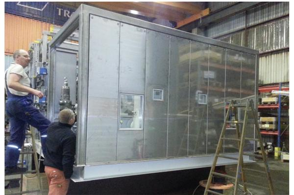
Test assembly of offshore enclosure
